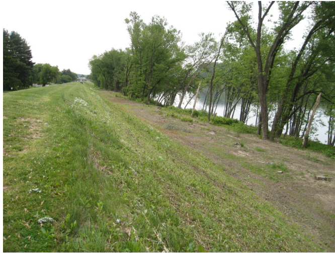
FIG. 2.1. River side of a levee with trees.
