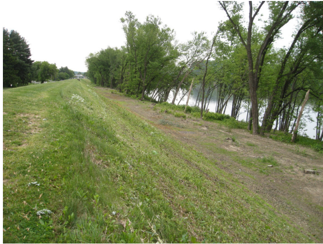
FIG. 2.1. River side of a levee with trees.
