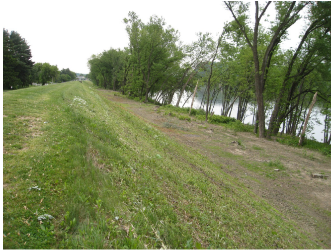
FIG. 2.1. River side of a levee with trees.
