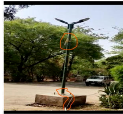
Fig. 4.7: Developed Prototype is installed at this pole of Sithauli Campus at ITM University, Gwalior, India. Initially Street Lights are in OFF Condition as the car is stationary object in this picture.
